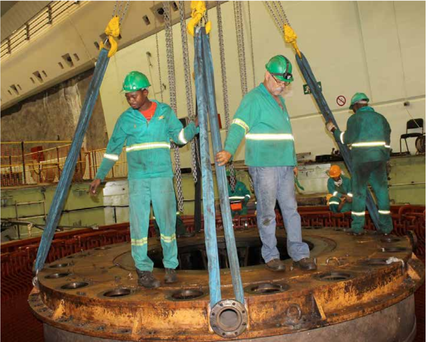
The removal of the turbine head cover.
